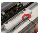
Place Cover over Hinge Knuckle with Grub Screws facing inwards towards Door Sash Open the door to expose the grub screws and tighten using a 2mm Allen Key
