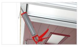
Apply the selected capping intumescent mastic in the (minimum) 10mm deep void on both sides of the doorset. Cap over the face of the any exposed packers.
