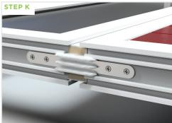
Apply 3 x beads of FSi Ltd Pyrocoustic Intumescent mastic on top of coupler strap before positioning the frame extension. Each bead must be a minimum of 120mm long and minimum of 8mm diameter.
