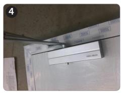
Secure the closing arm and cover plate. Check operation and adjust the closing forces to meet the application.
