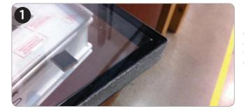
When handling glass, care must be taken to ensure the factory fitted fire tape (Intumescent) is not damaged during the glazing process.
