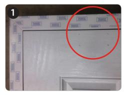
Identify the pre-drilled pilot holes on the leaf and frame
