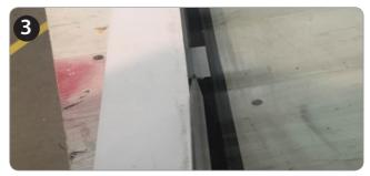
Using a rubber mallet, fix the glazing bead in place to secure the DGU. NB/ The glass is fragile and extra care must be take when glazing a fire door top light.
