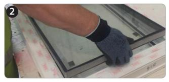
Lower the glass into the frame, making sure the intumescent tape is not damaged, and the glass sits squarely on all of the glazing clips.
