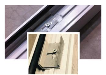
With the glass removed, you will be able to see the glazing clips that have been installed in the factory. The locking clip is a two part system.
