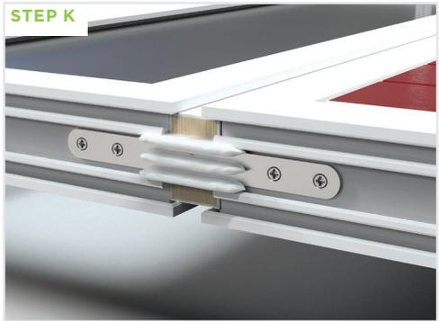
Apply 3 x beads of FSi Ltd Pyrocoustic Intumescent mastic on top of coupler strap before positioning the frame extension. Each bead must be a minimum of 120mm long and minimum of 8mm diameter.
