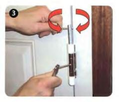
When in position secure the socket screw and replace the covers.
