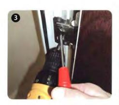
Secure the screws in the side plate.
