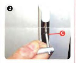
With a 4mm allen key loosen the socket screws (C) by about 1/3 of a turn
